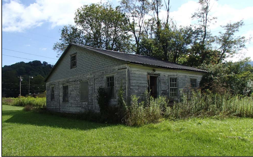
Figure 23: former Mabel School, southwest corner
