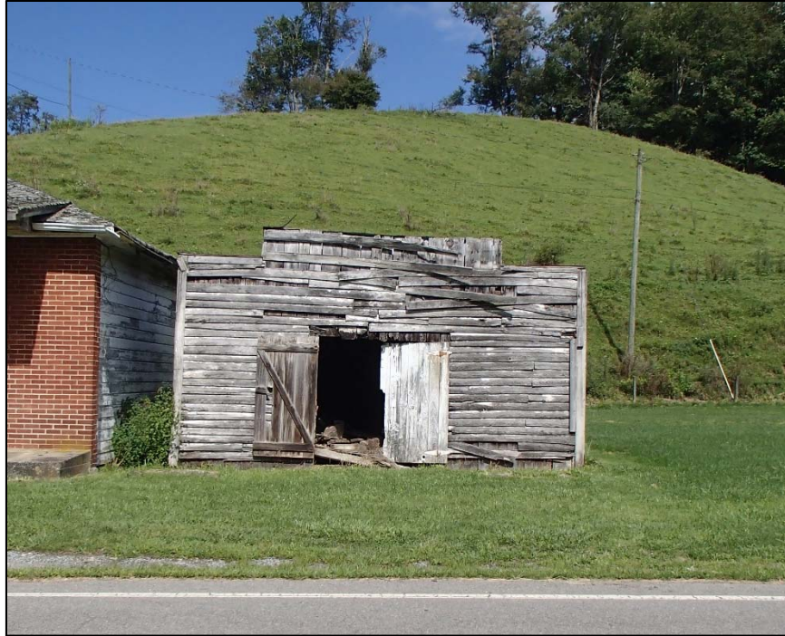
Figure 50: Mast Store Storage Building 1, east elevation
