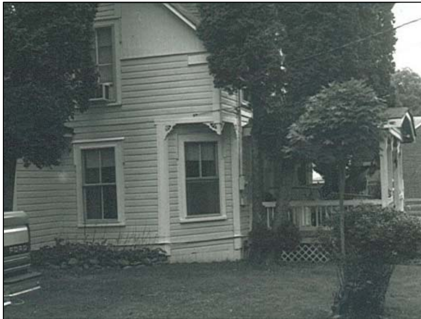
Figure 44: Jack Campbell House, northwest corner, 1978 survey photograph
