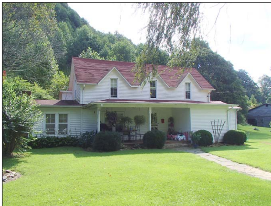
Figure 4: Eli and Louise Church House, west elevation
