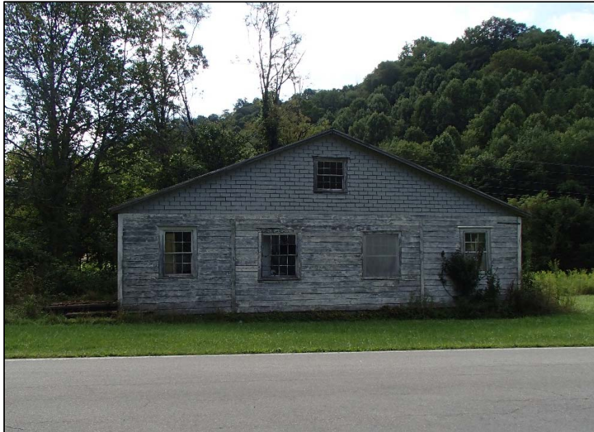
Figure 24: former Mabel School, west elevation
