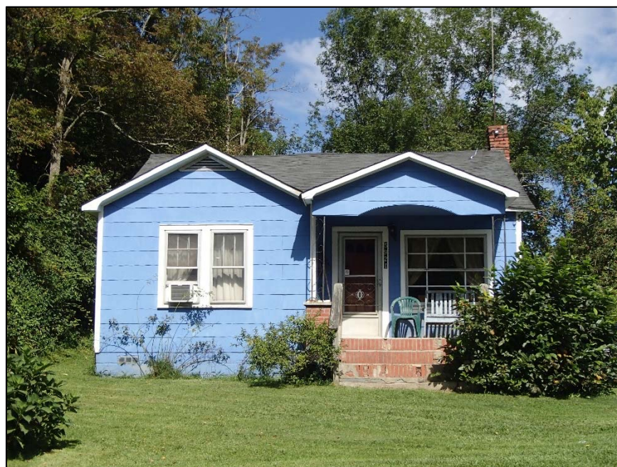
Figure 55: Eli and Minnie Oliver House, east elevation
