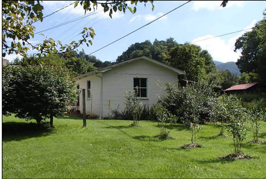
Figure 21: Younce House, concrete block outbuilding, south elevation
