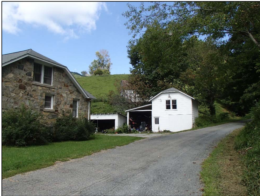
Figure 48: Bert and Hazel Mast House, garages
