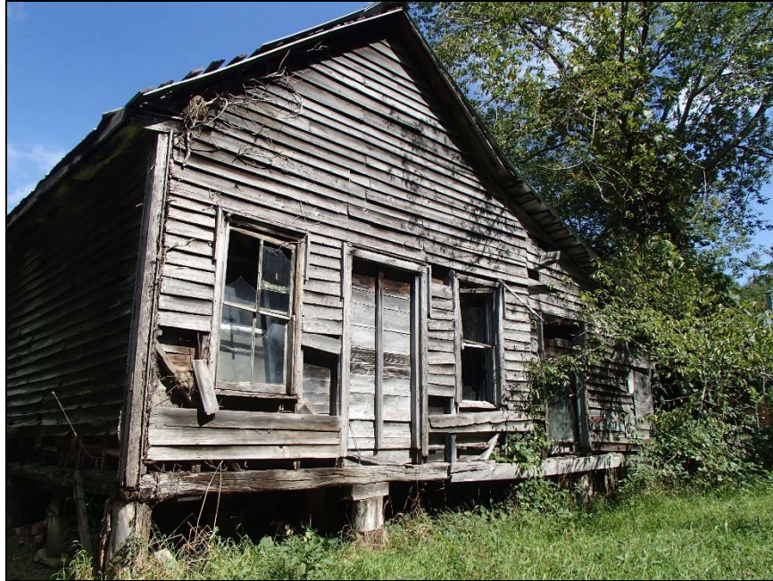
Figure 14: Mabel Store and Post Office, east elevation (original front)
