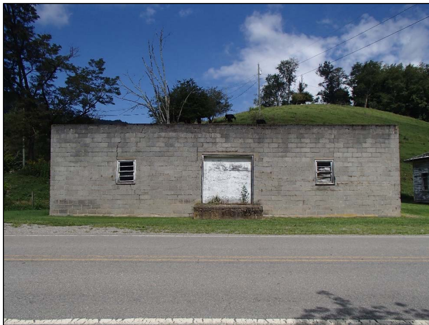
Figure 54: Mast Store Storage Building 2, east elevation
