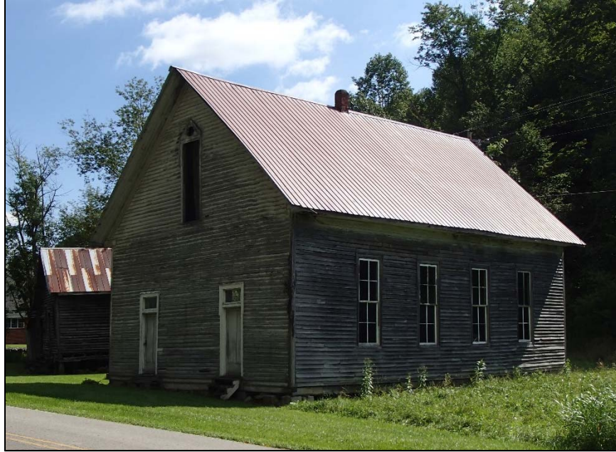
Figure 9: former Mabel Methodist Church, southwest corner
