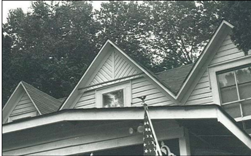
Figure 43: Jack Campbell House, west elevation detail, 1978 survey photograph
