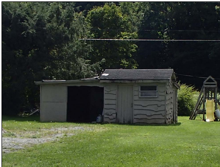
Figure 22: Younce House, wavy-siding outbuilding, west elevation
