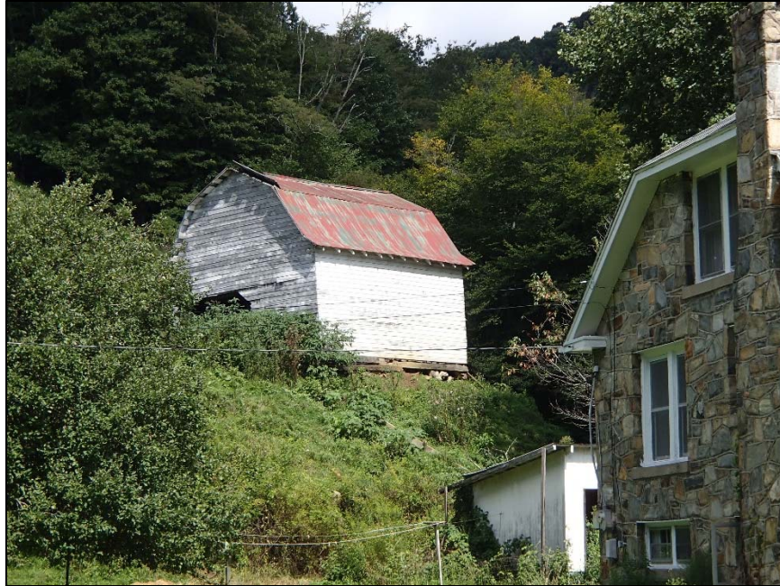
Figure 49: Bert and Hazel Mast House, barn
