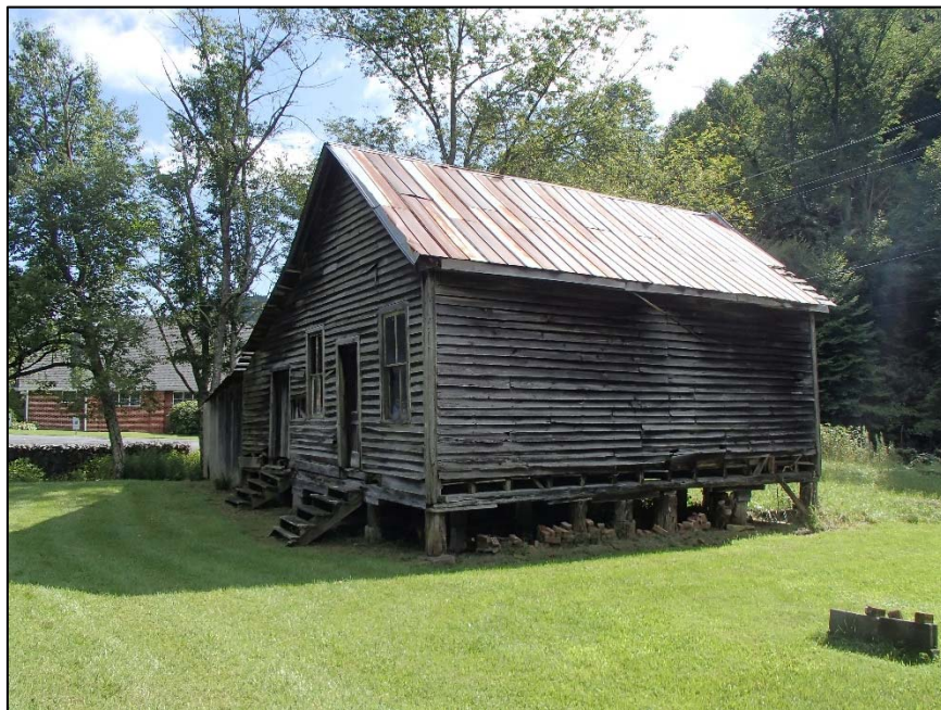
Figure 15: Mabel Store and Post Office, south elevation
