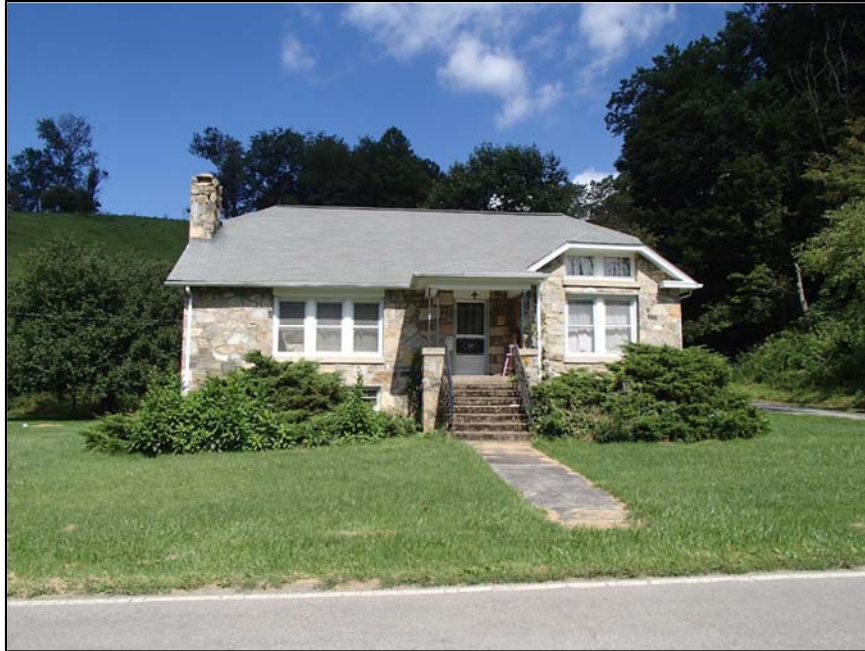
Figure 45: Bert and Hazel Mast House, east elevation
