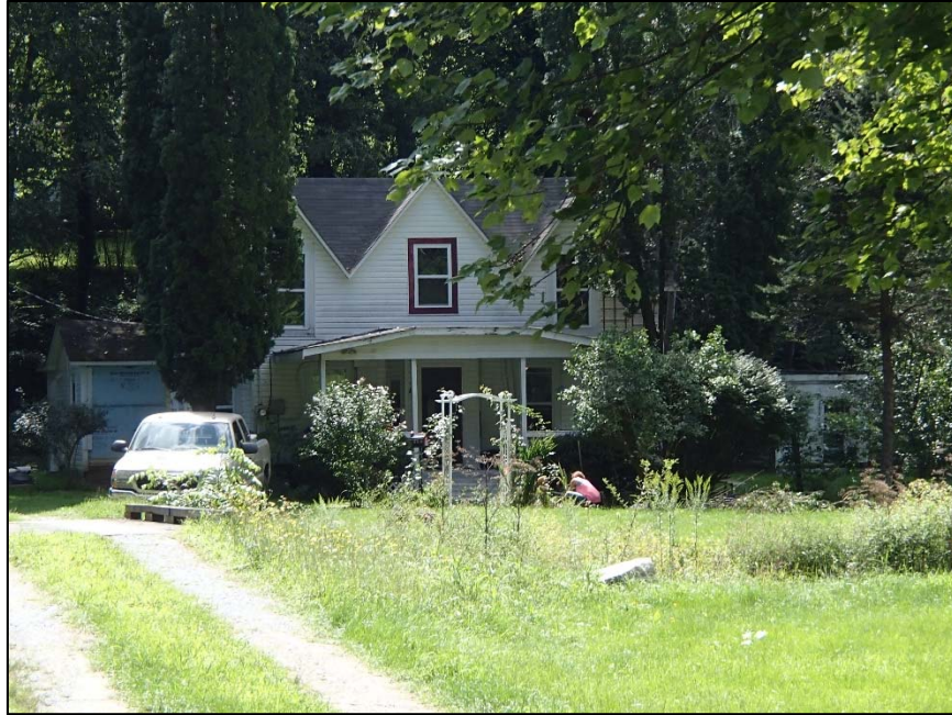
Figure 41: Jack Campbell House, west elevation
