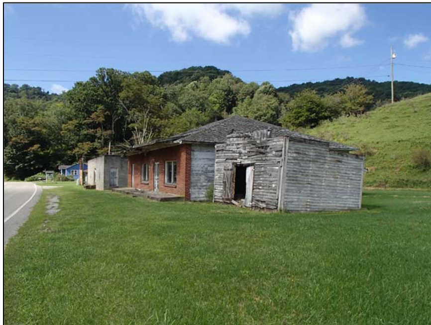
Figure 51: Mast Store Buildings, showing north elevation of Storage Building 1
