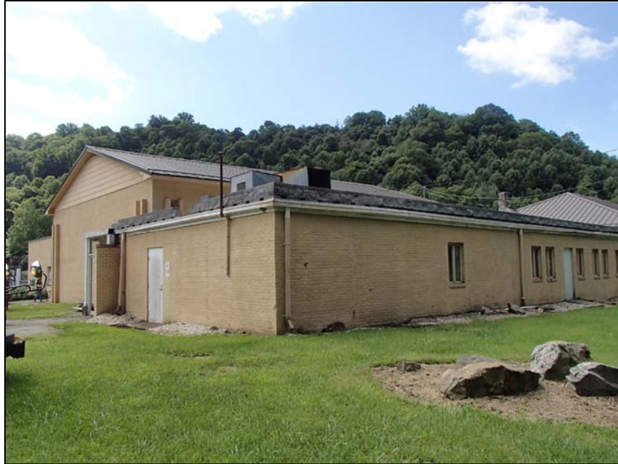
Figure 30: Mabel School, northwest corner
