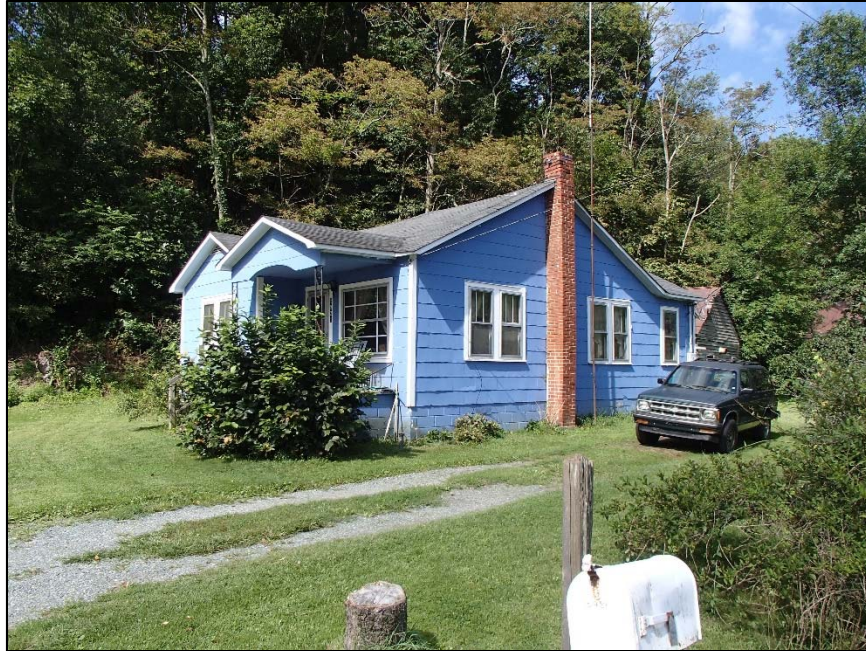
Figure 56: Eli and Minnie Oliver House, northeast corner
