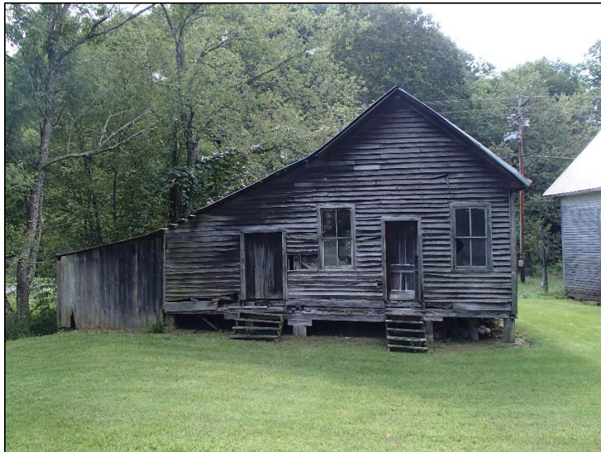
Figure 13: Mabel Store and Post Office, west elevation (original rear)
