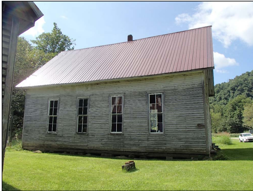
Figure 12: former Mabel Methodist Church, north elevation
