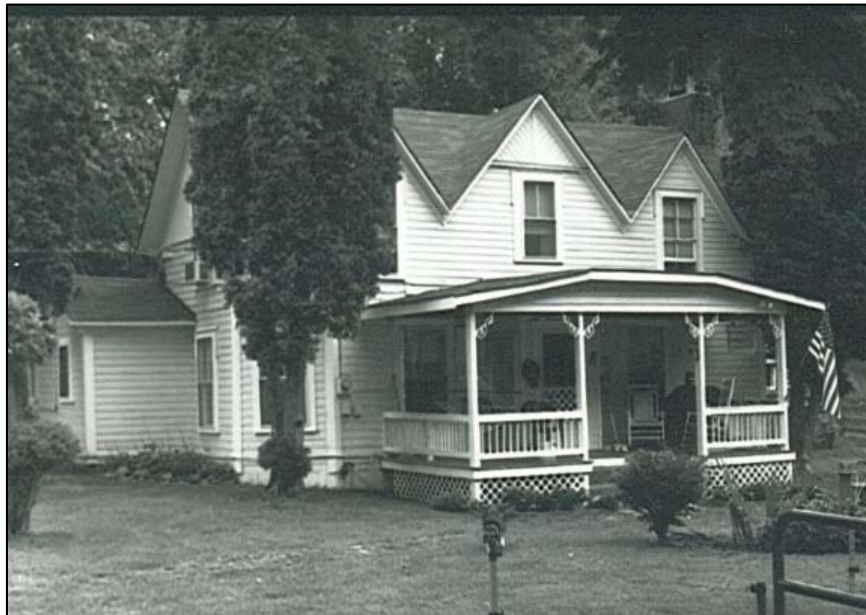
Figure 42: Jack Campbell House, west elevation, 1978 survey photograph
