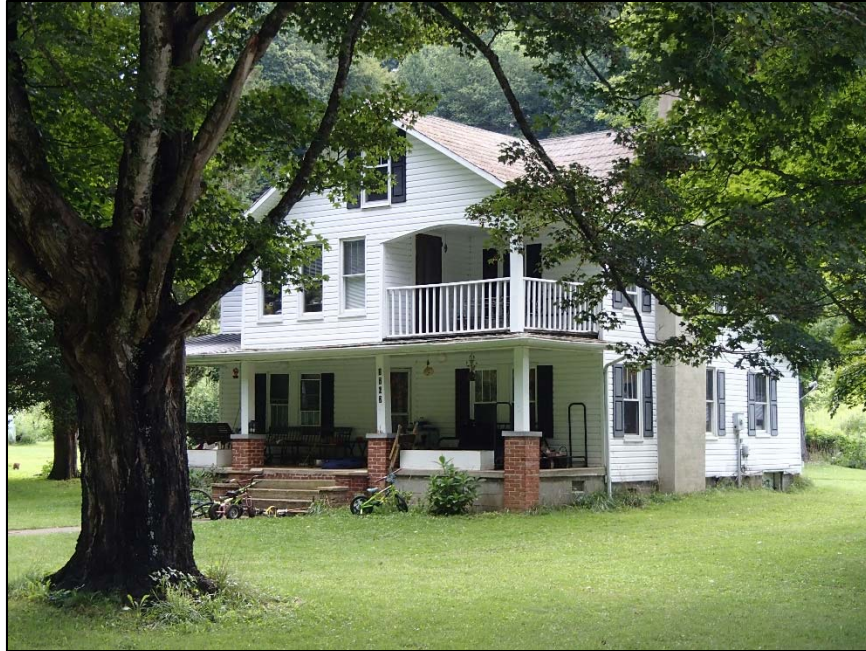
Figure 32: Grant Lawrence House, west elevation
