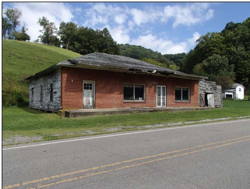
Figure 53: Mast Store, southeast corner
