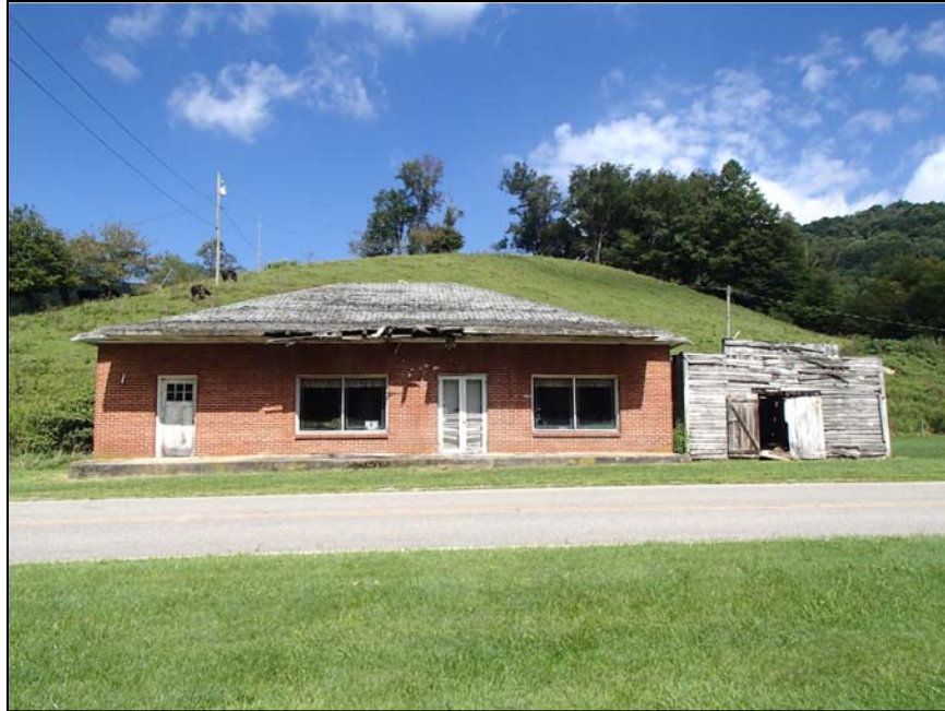
Figure 52: Mast Store, east elevation
