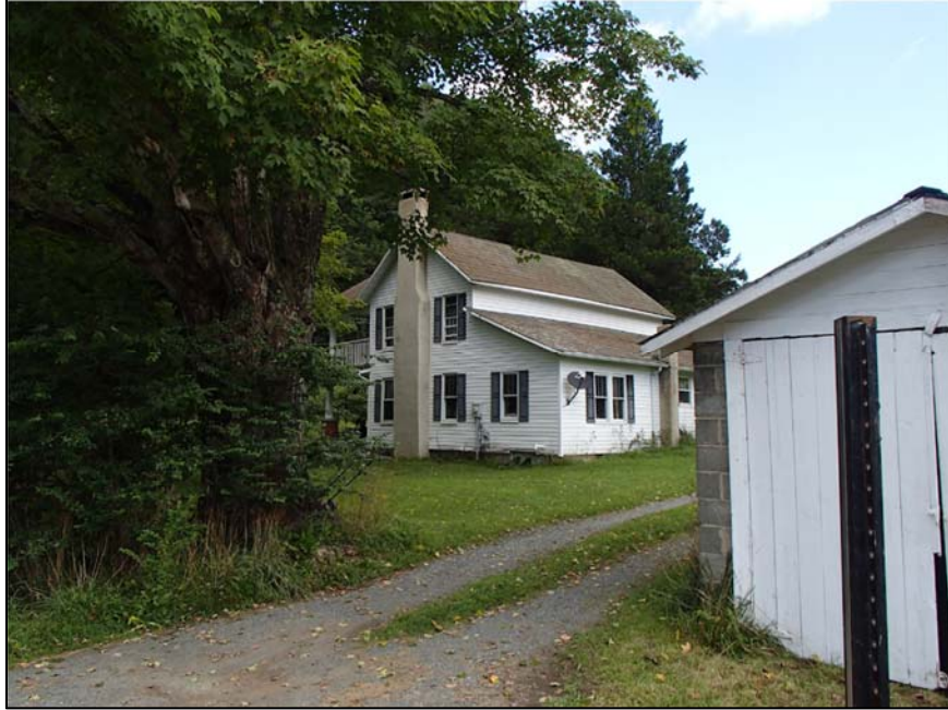
Figure 34: Grant Lawrence House, southeast corner
